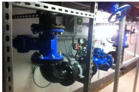
PRV Installation
